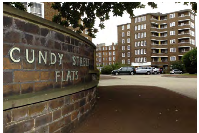
Cundy Street flats before demolition
