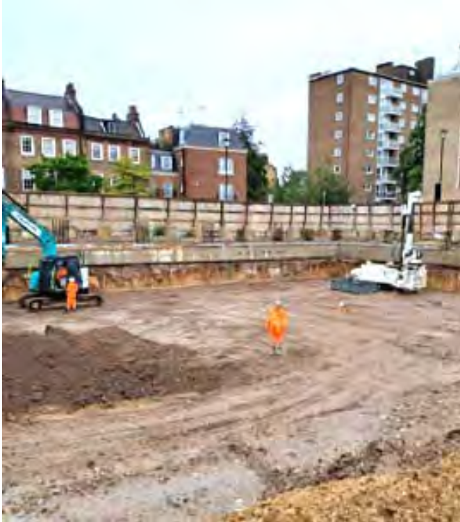
Cundy Street works
