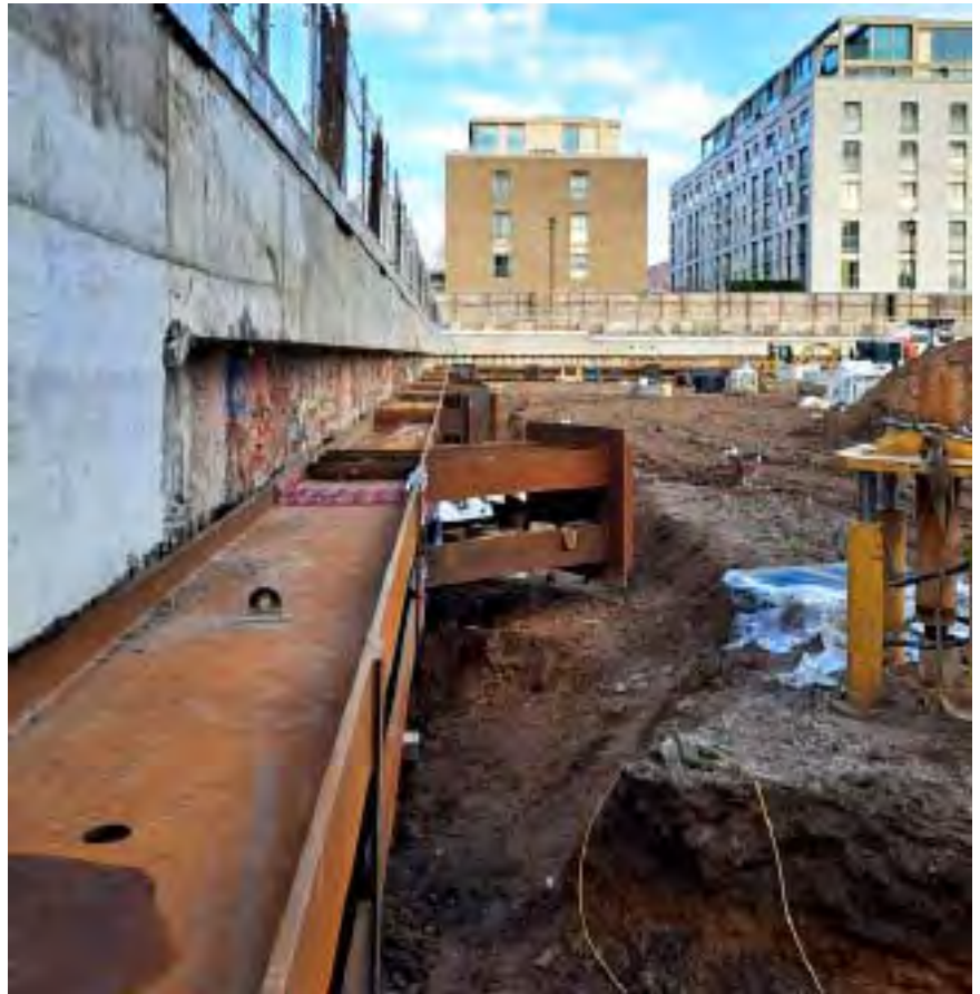
Cundy Street works
